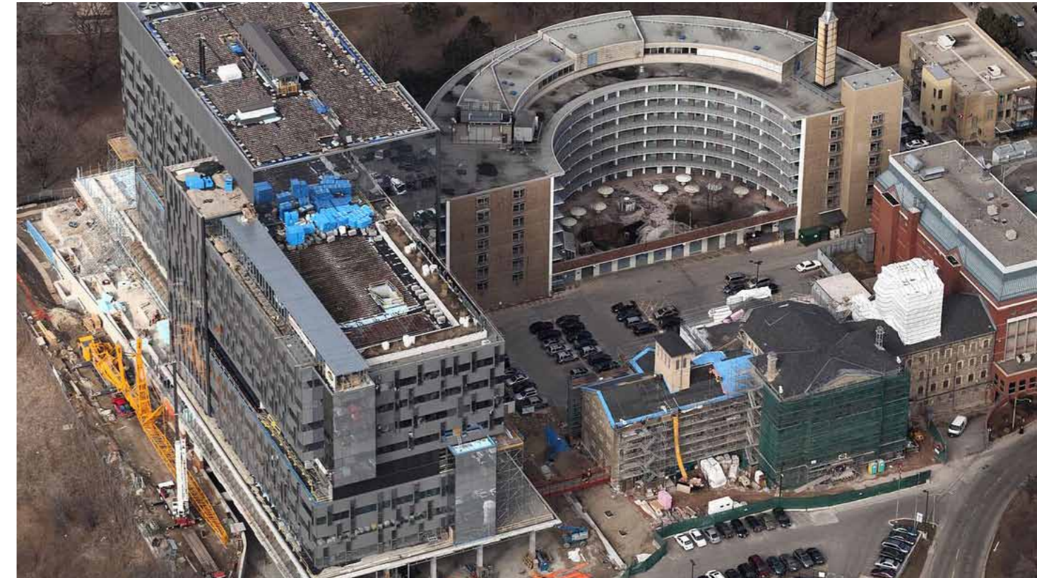
Aerial view of Bridgepoint Hospital redevelopment
