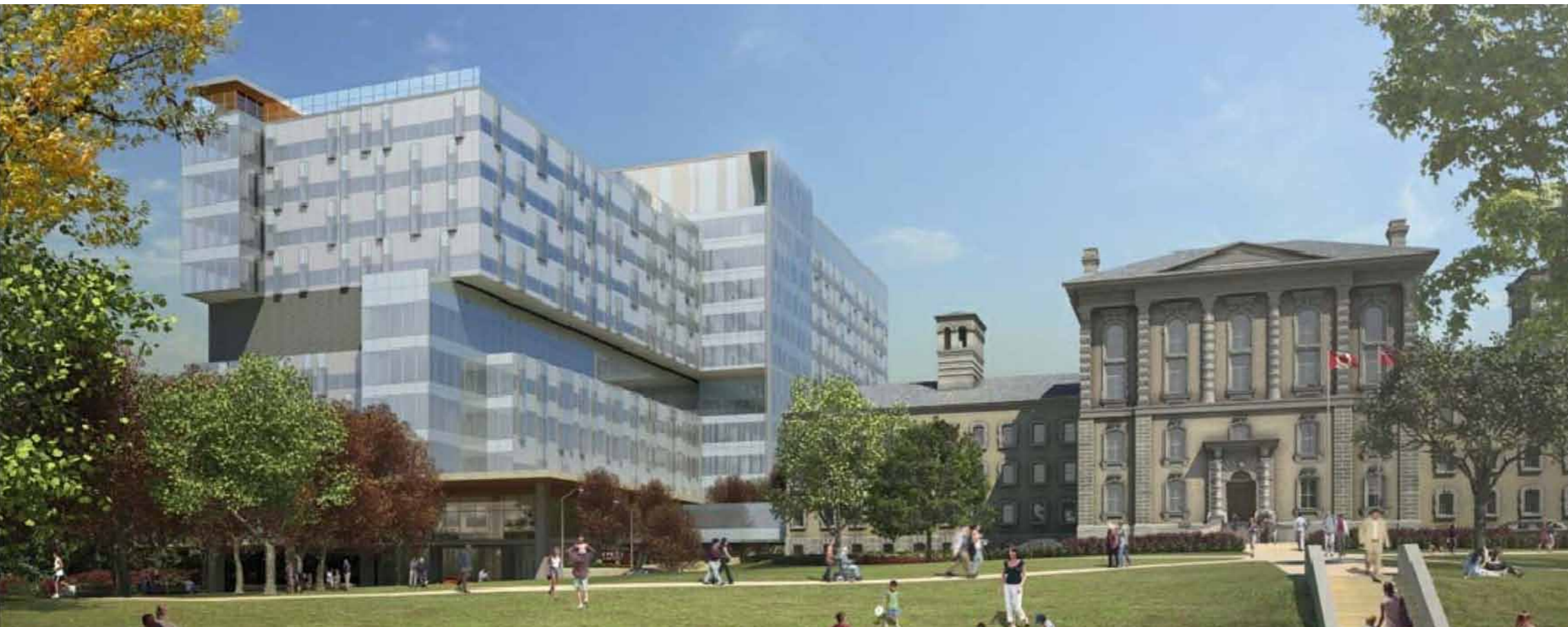
Bridgepoint Hospital, view from south-east
