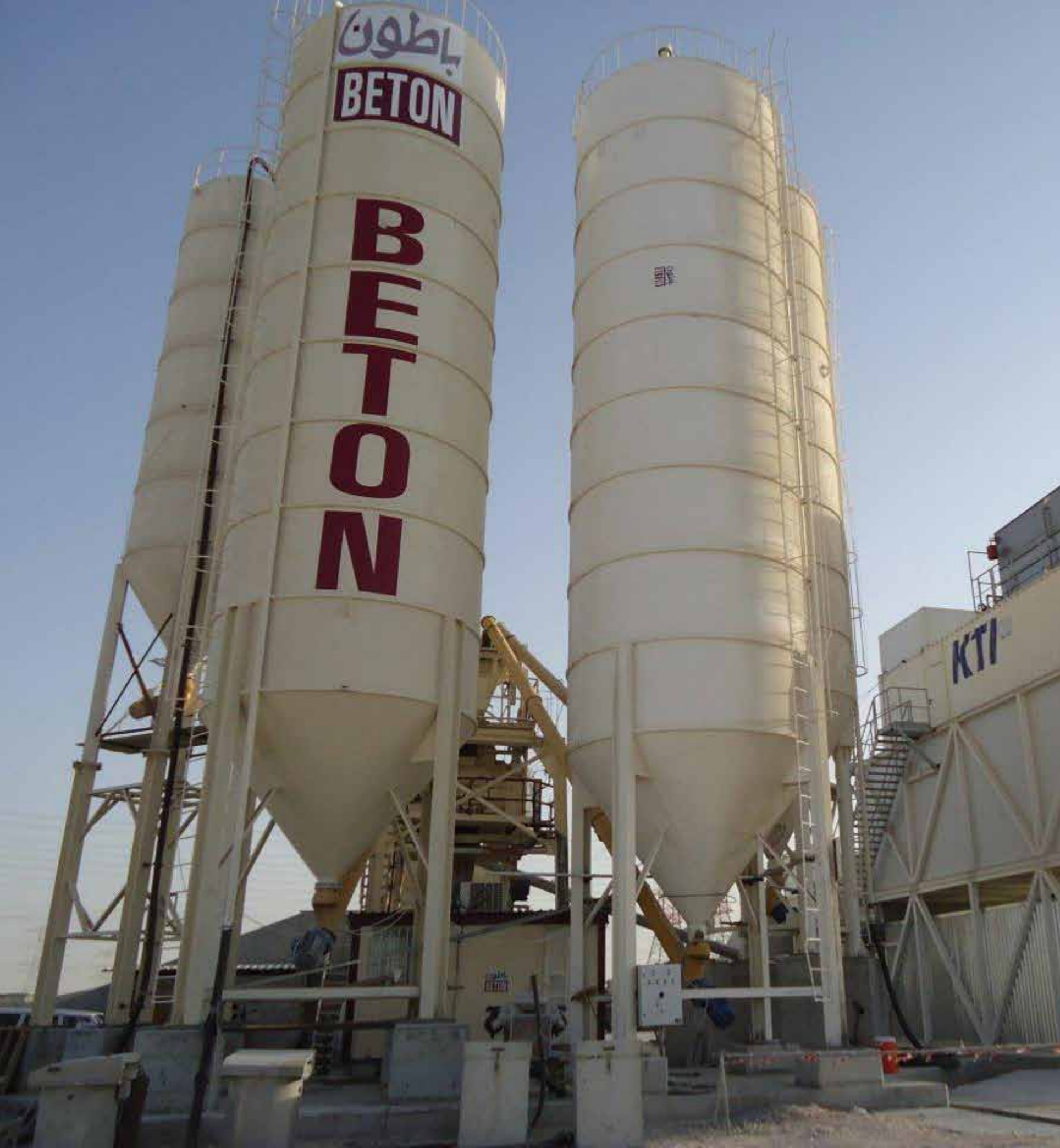
Batching plant and KTI ice and chiller plant
