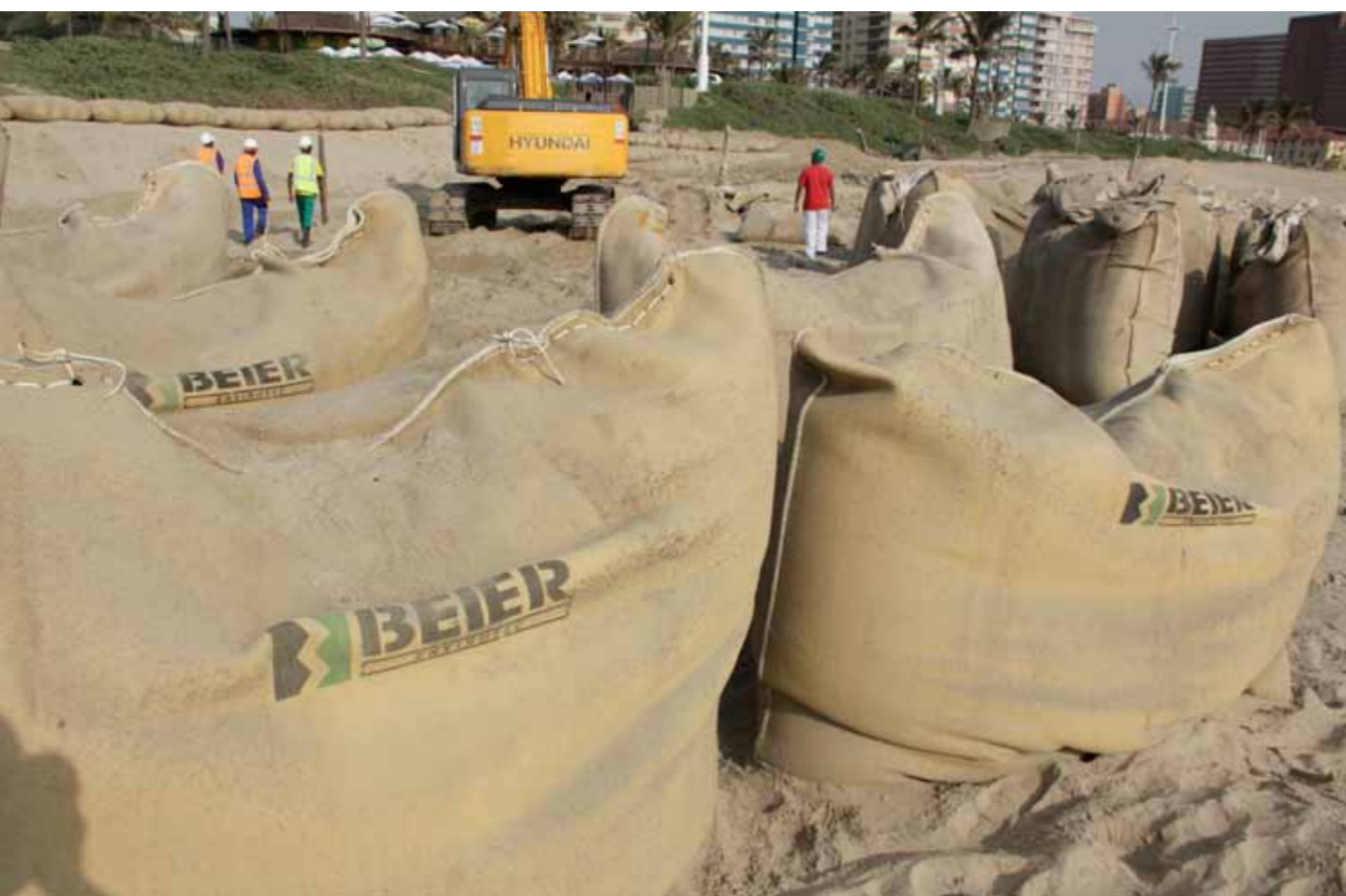
Beier products on site
