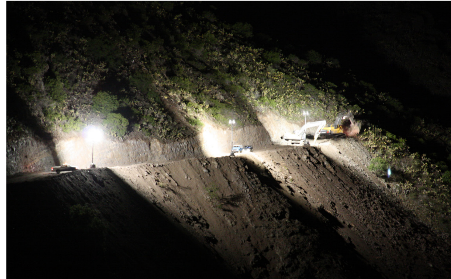
Working at night on the haul road
