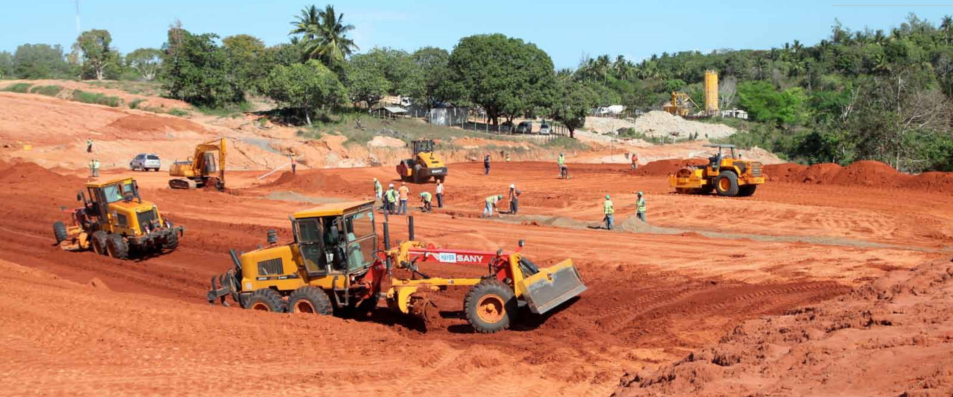
Water storage dam - central embankment under construction
