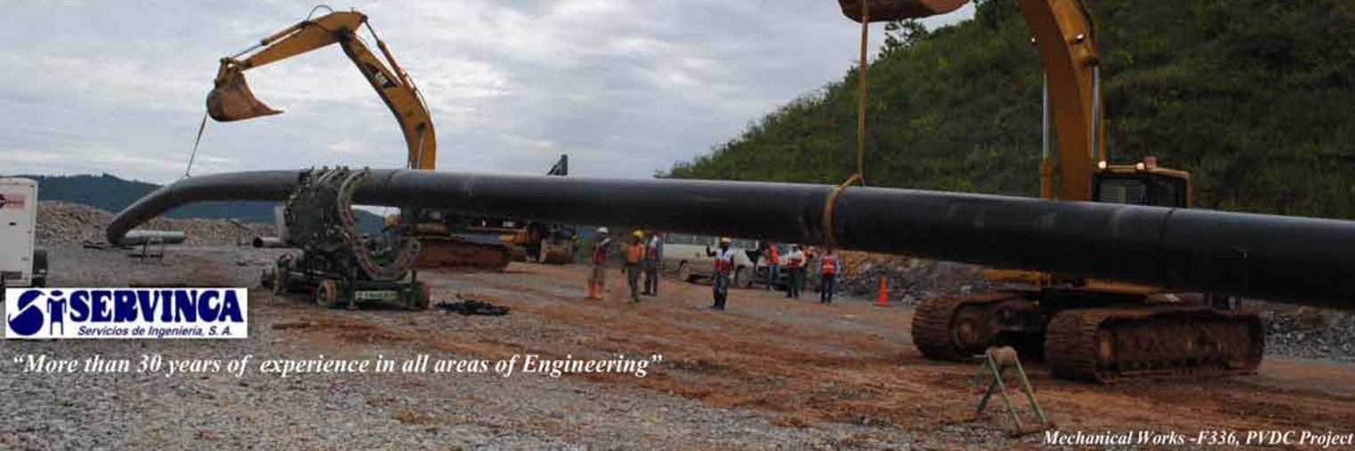
HDPE Piping Thermofusion
