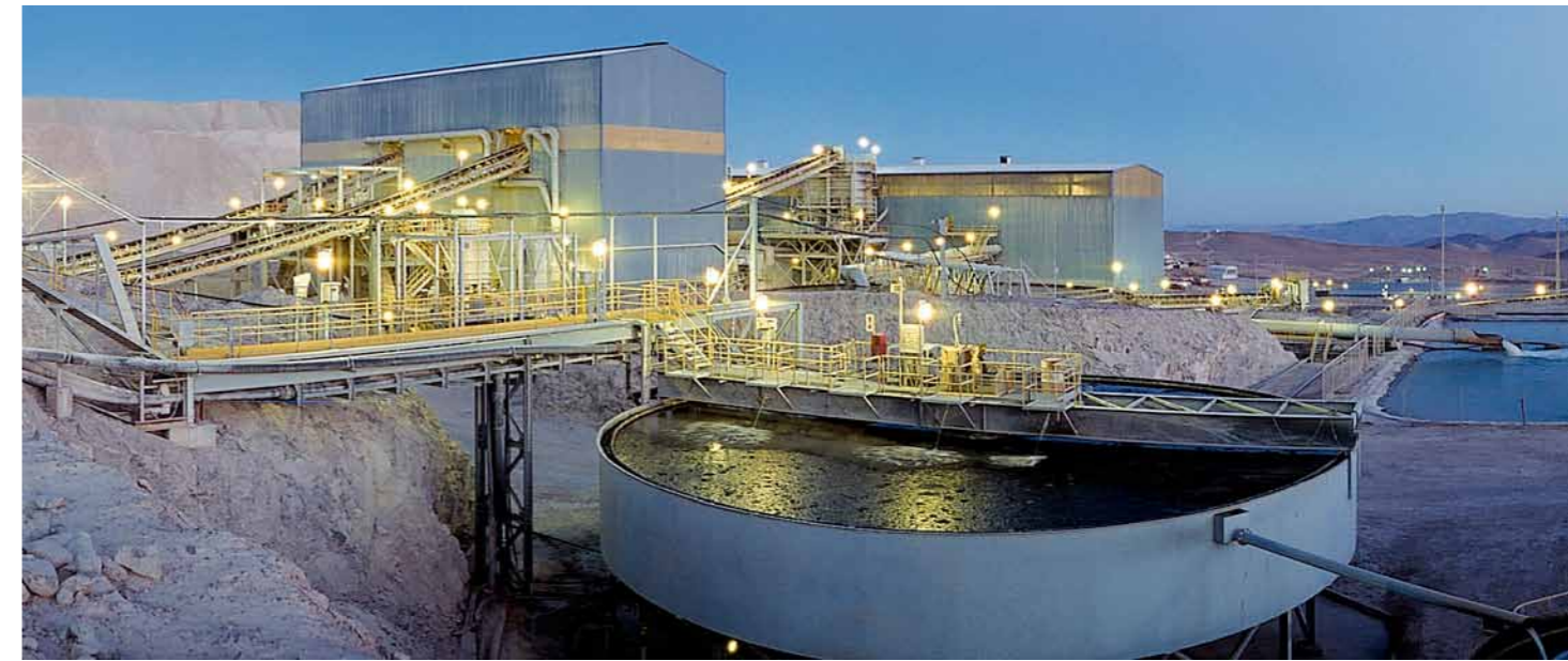
Zaldivar copper process facility
