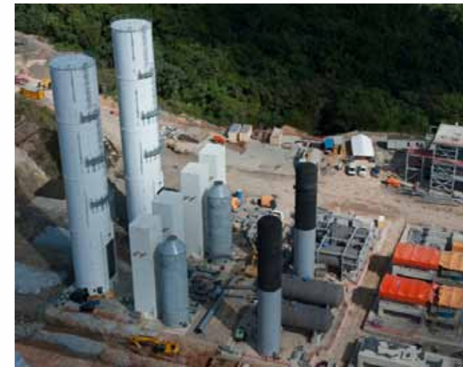
Steam and oxygen are injected into the autoclaves to oxidize the ore
