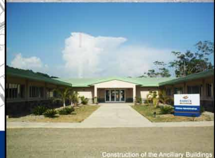
Construction of the Ancillary Buildings
