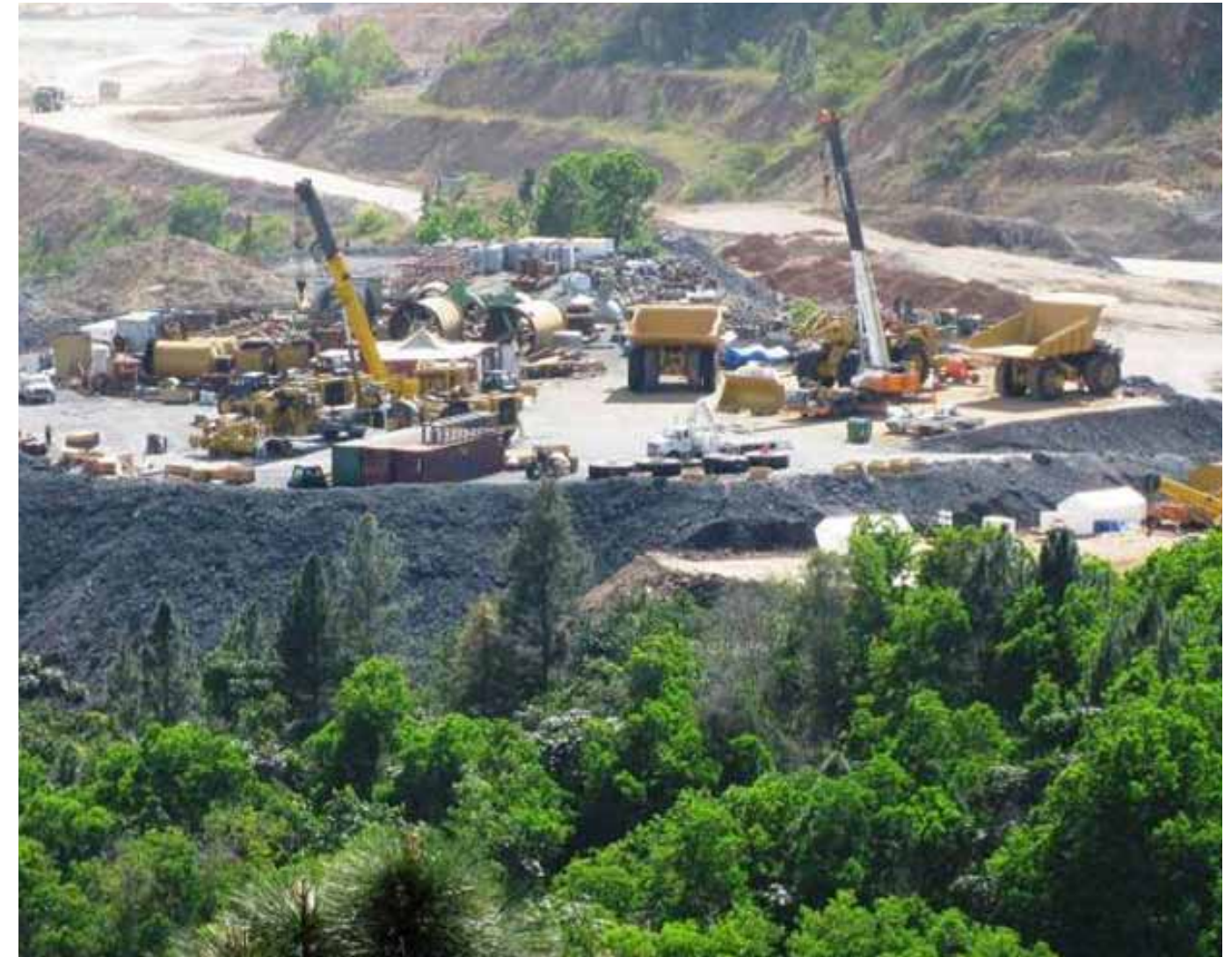
Mine equipment being assembled at Pueblo Viejo
