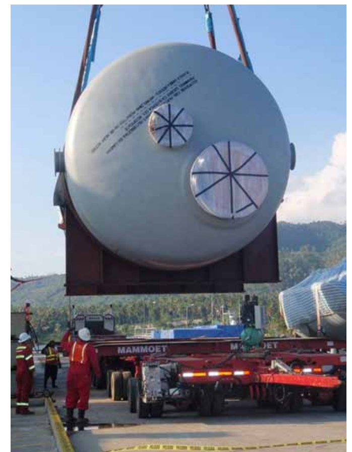
A flash vessel for the pressure oxidation process is off loaded
