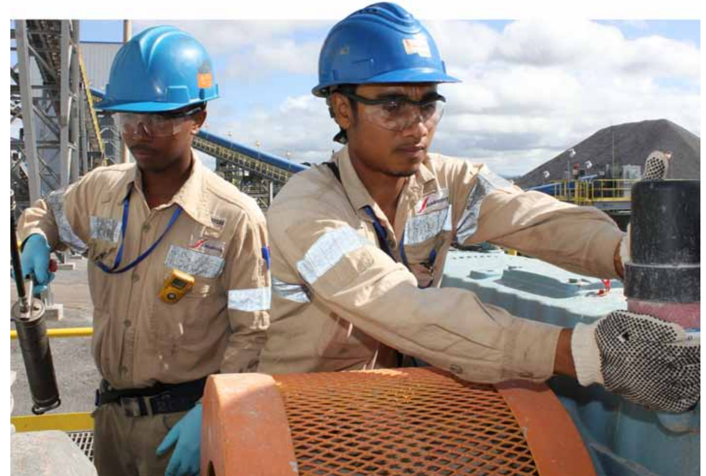
Maintenance at the refinery
