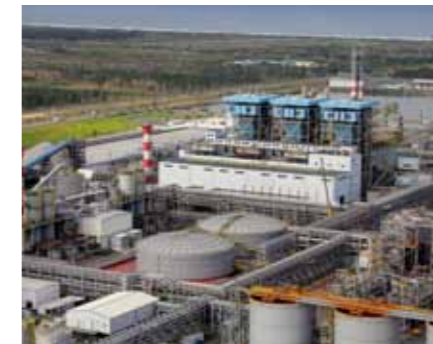
Ambatovy has now entered the operational phase
