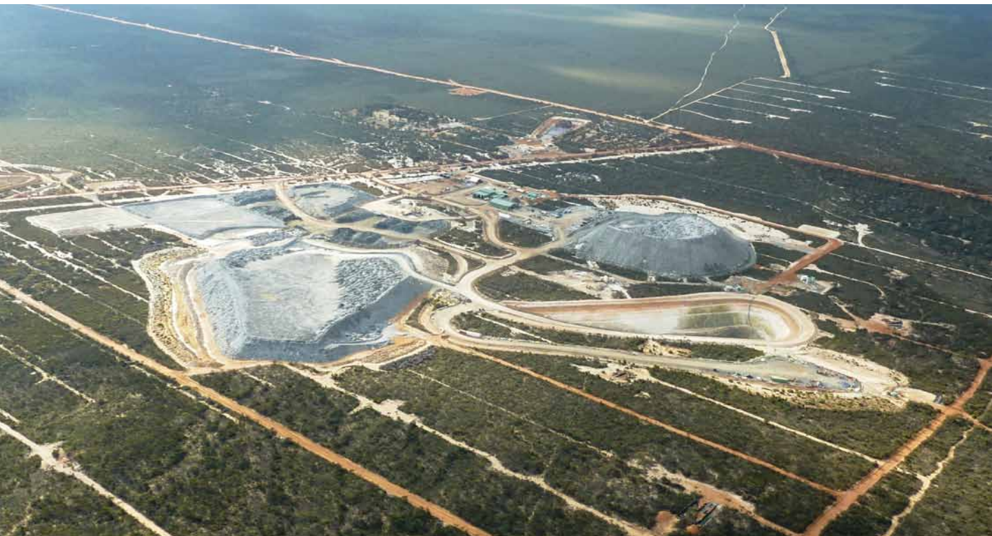
The Flying Fox mine uses ATMOS Global technology to determine optimal allocation of dust management strategies
