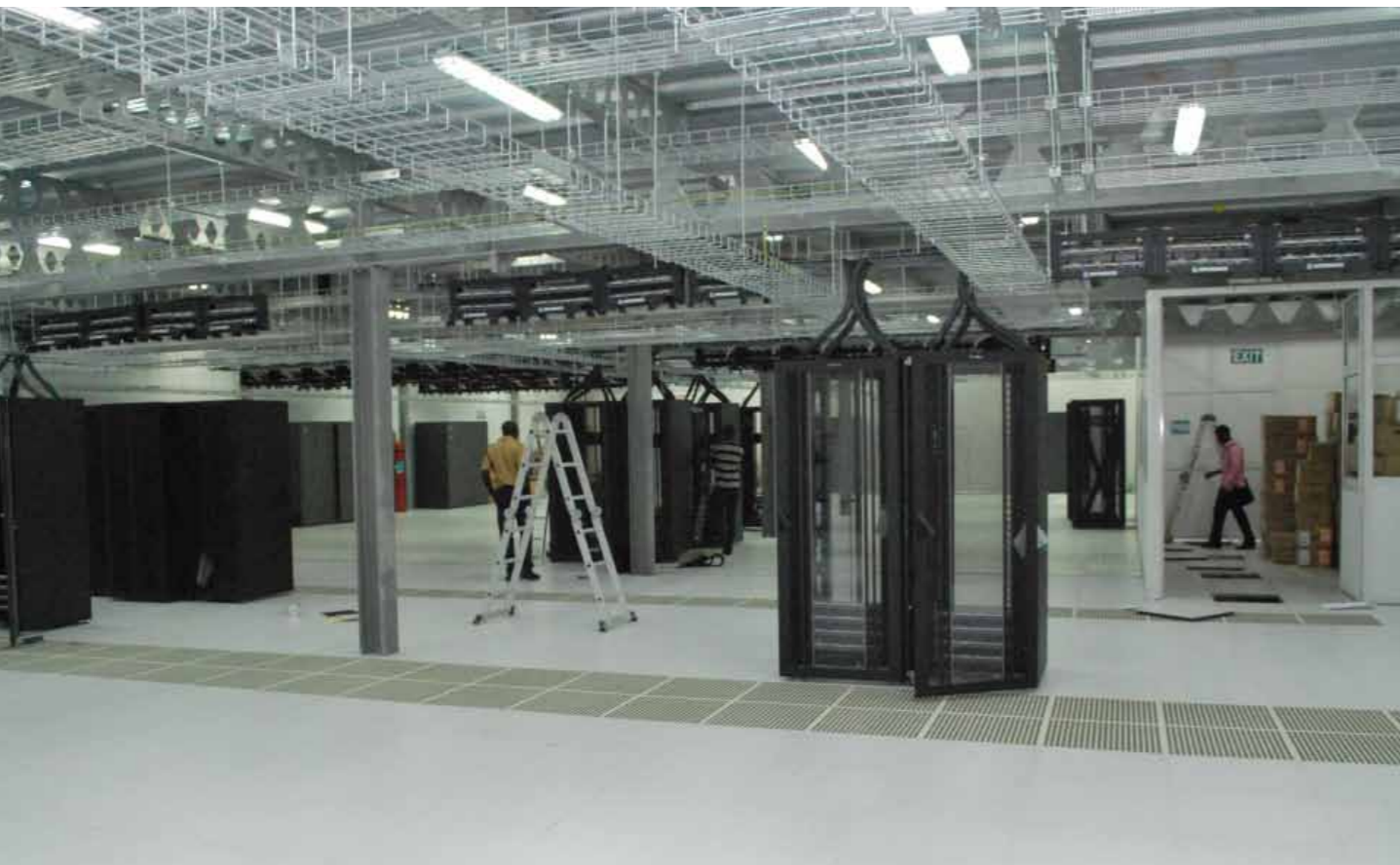
Inside the data centre during installation of the server racks
