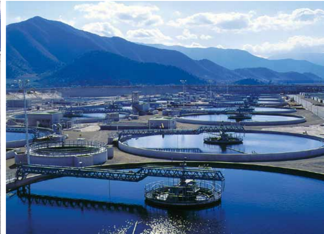
View of La Farfana sewage treatment works in Chile
