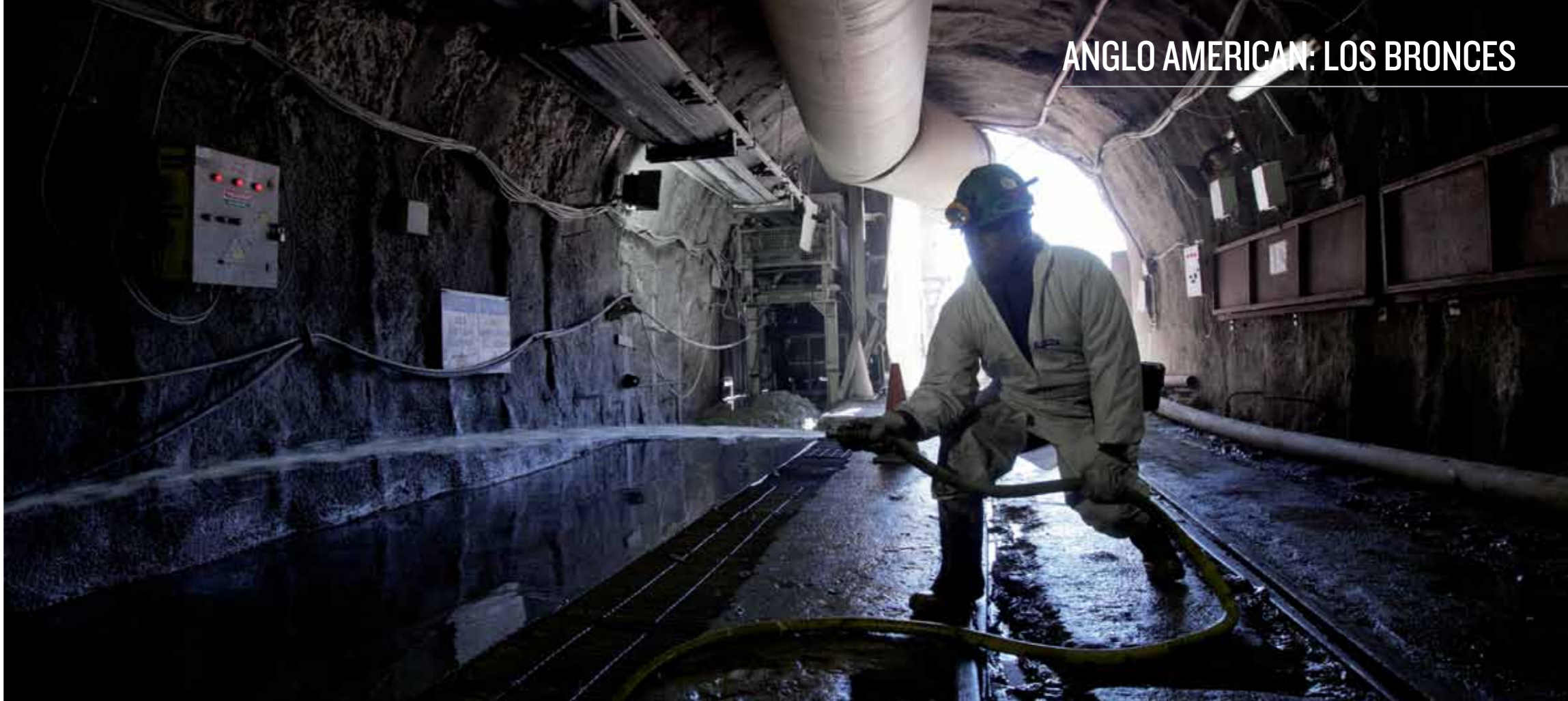
Routine cleandown of the exploration access tunnel
