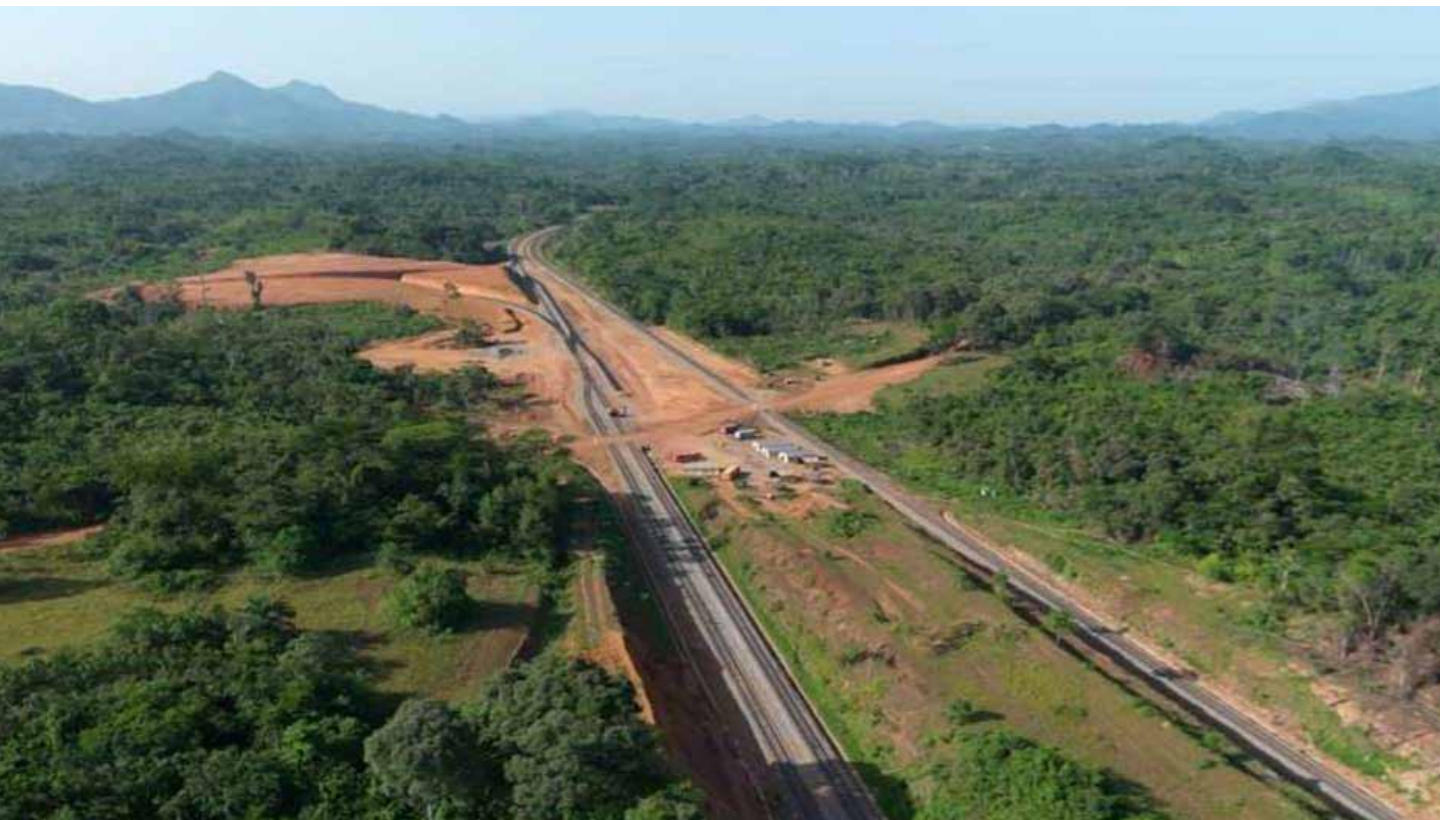
Upgraded railway line linking Kokoya project to Buchanan Port in Liberia
