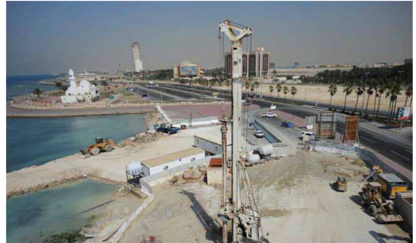
Aerial view of piling works
