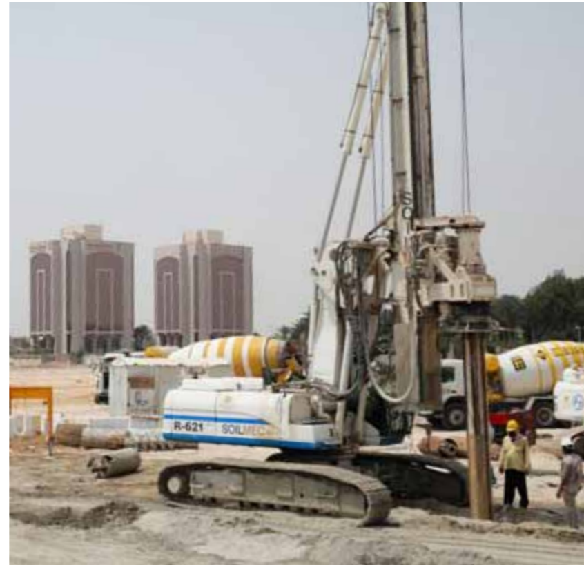
Piling works in progress
