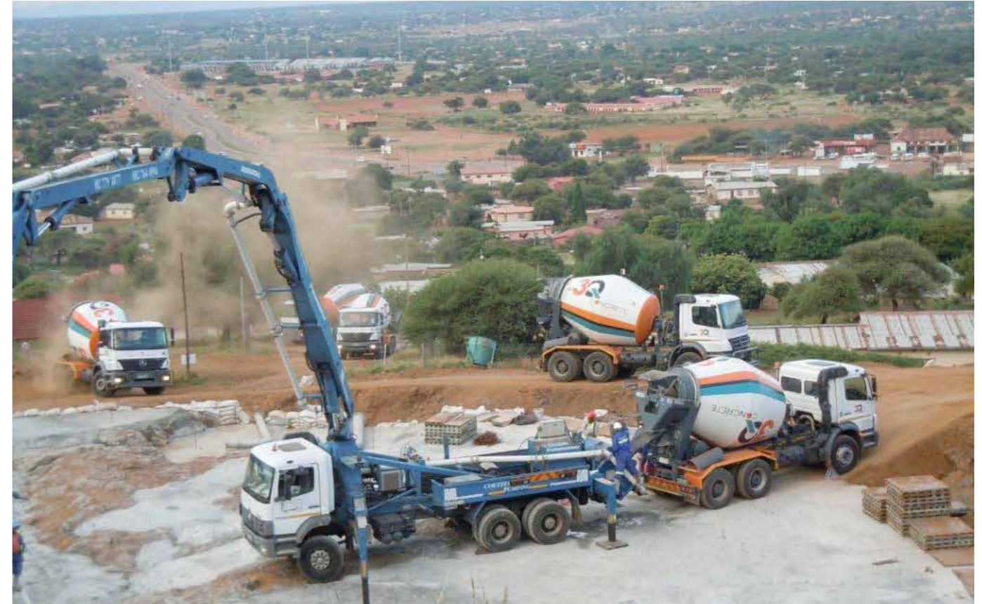
3Q Concrete produce both normal and customised mix designs
