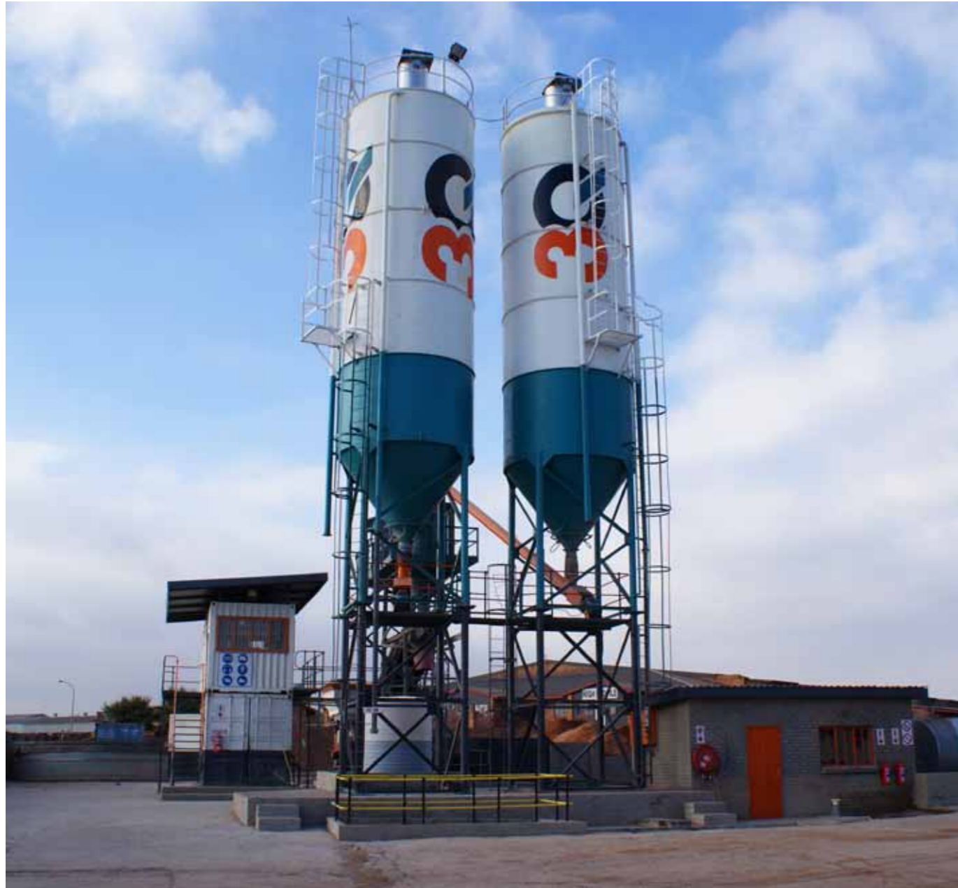
3Q Concrete aims to open three new batching plants in 2013
